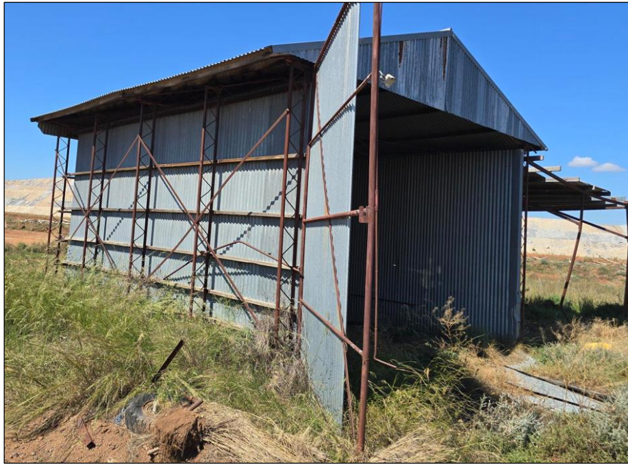
Figure 36 - Shed demolished in 2025
